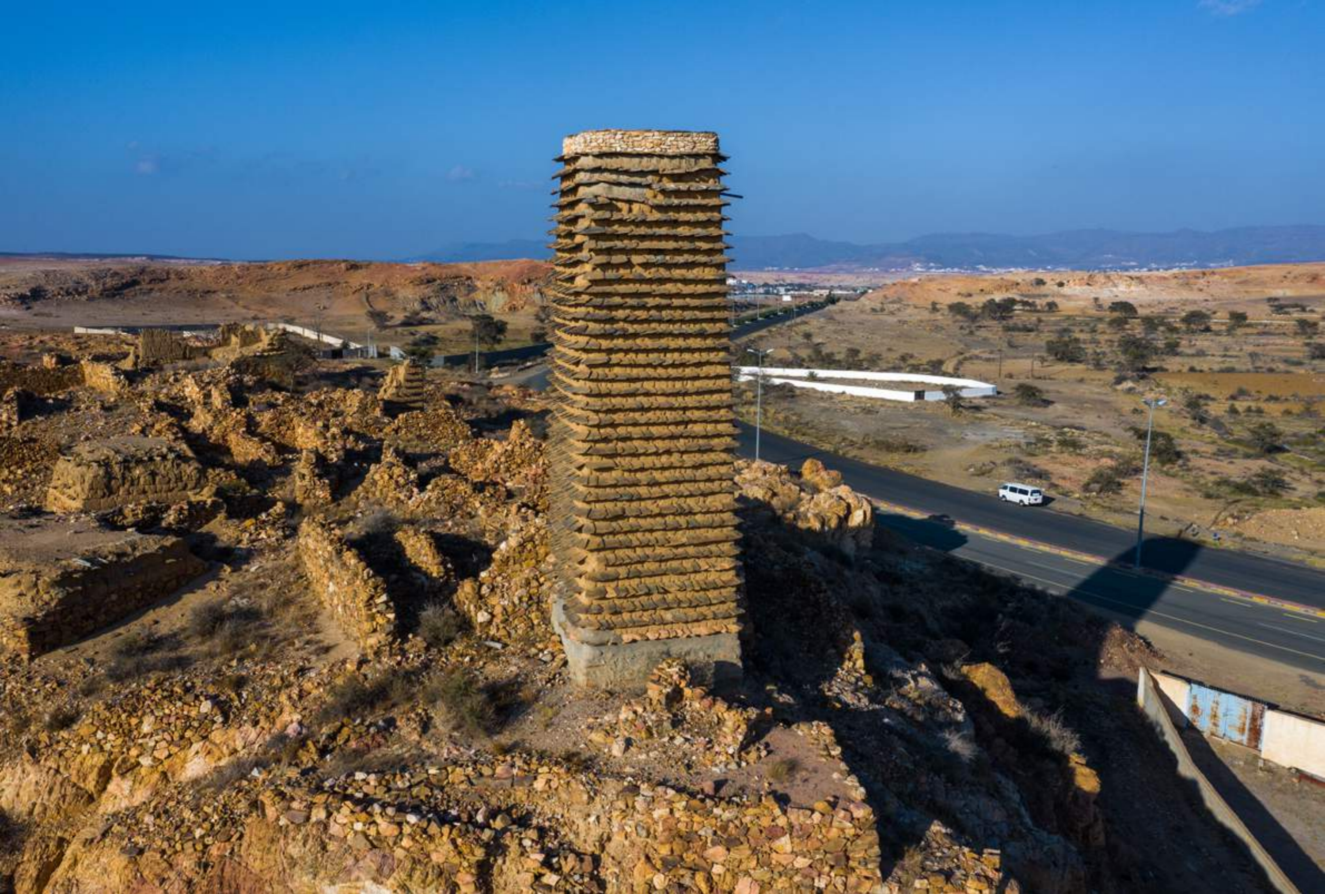
A stone and mud watchtower made of slates standing in the Asir province of Saudi Arabia. These watchtowers had two purposes: to monitor neighboring enemies and to keep harvests safe in this arid area. Nowadays, they have become the symbol of Asir province and can be seen all along major roads.
